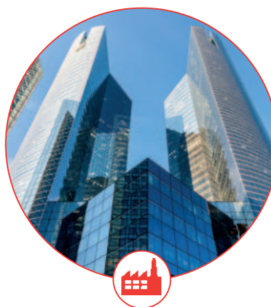
INDUSTRY AND TERTIARY BUILDINGS
