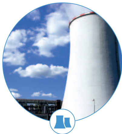
ELECTRICAL POWER GENERATION
